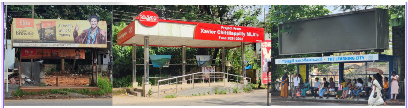
Figure 7. Infrastructural hierarchy identified in the study. Left: an old shelter on peripheral routes, lacking basic amenities. Centre: the only existing accessible stop in the dataset. Right: the latest type of bus stop infrastructure seen in the urban core, representative of the UNESCO programme.
