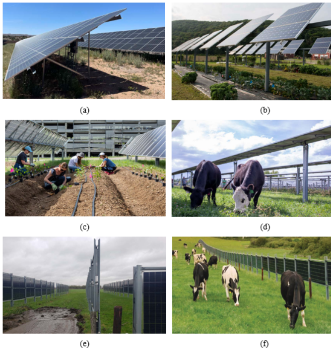
Figure 9. Different photovoltaic configurations for agrivoltaic systems – (a) Fixed tilt continuous, (b) Fixed tilt partitioned, (c) Single axis tracking without elevated panels, (d) Single axis tracking with elevated panels, (e) and (f) vertical bifacial. Source: Staie and Mirletz [40].
